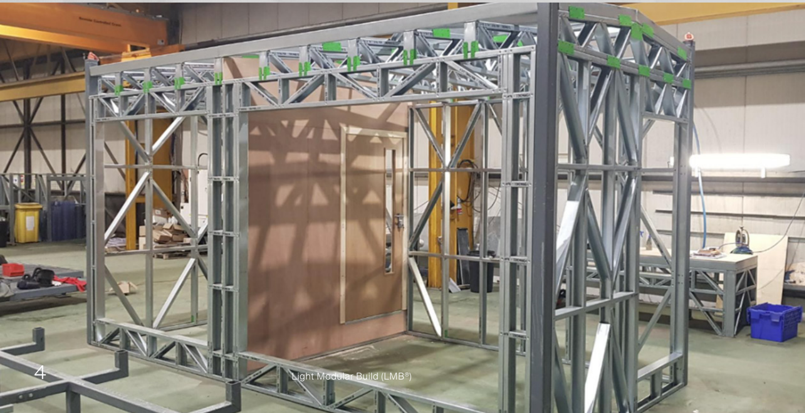
Image below: Fabrication of LMB® at RSE's Muir of Ord facility.
