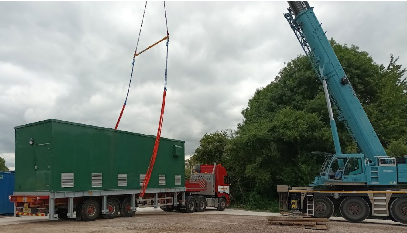
Below: DfMA crane lifted at site
